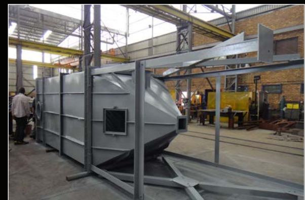
Fabrication of baghouse
