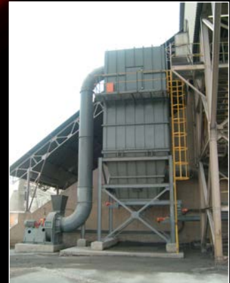
Bag filter Installation
