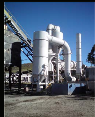
Wet Scrubber Installation
