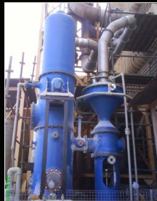
Wet scrubber installation
