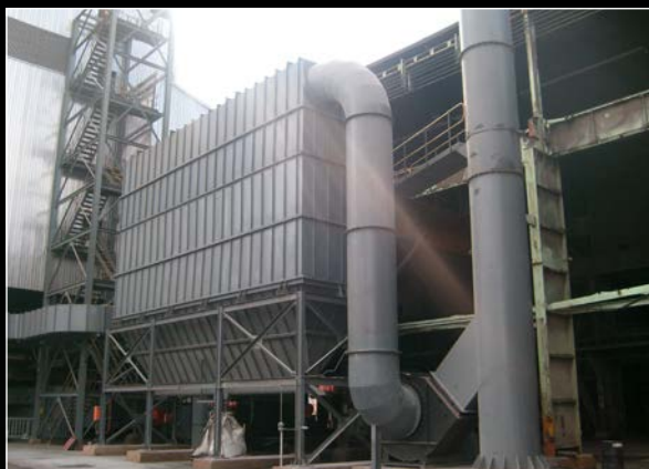
Bag Filter installation
