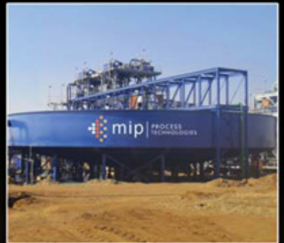
26m \phi Thickener in operation
