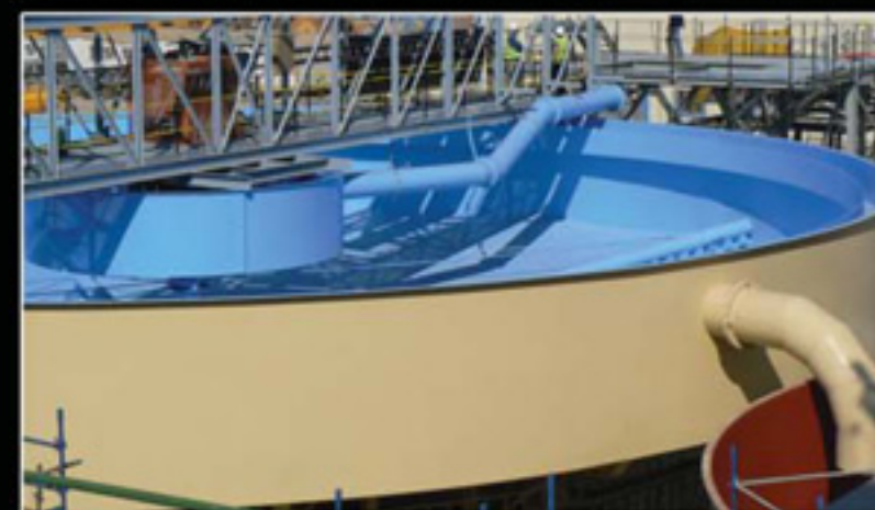
26m \phi Thickener installation
