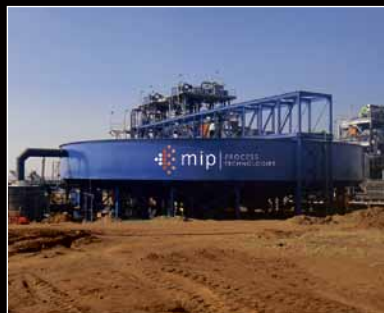
26mØ Thickener in operation
