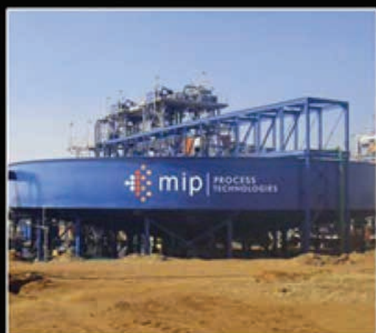
26m \phi Thickener in operation
