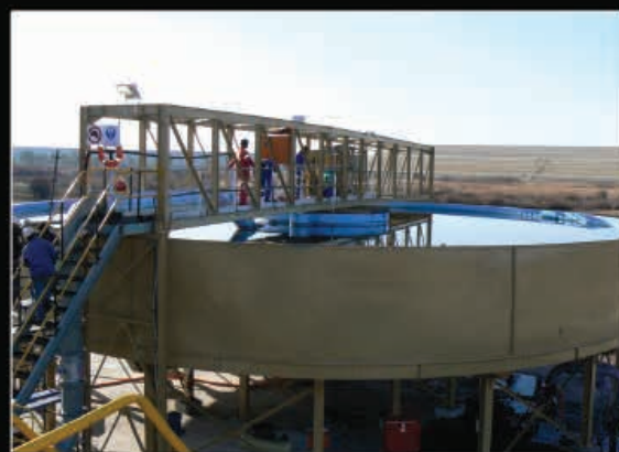
21m \phi Thickener from bolted design
